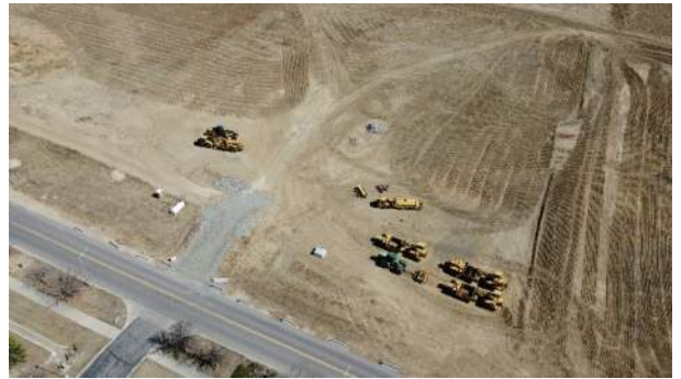
Construction Entrance and Equipment Storage - Northeast
