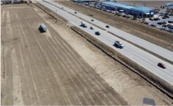
HWY 119 Ditch - Southeast
