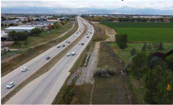
HWY 119 Ditch Outfall - West
