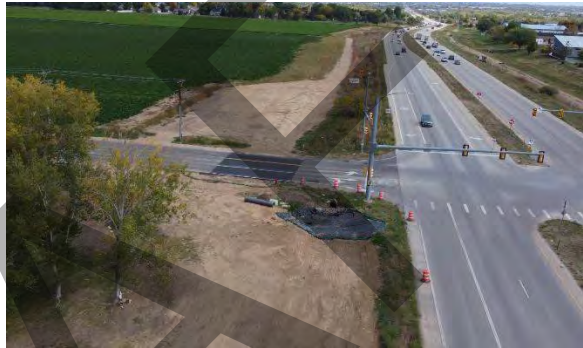
HWY 119 Ditch - East
