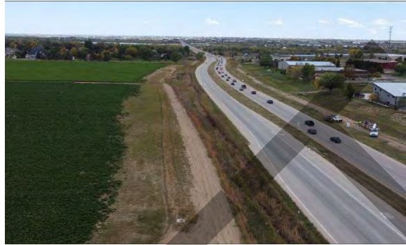
HWY 119 Ditch Outfall - East
