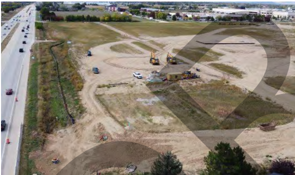
Commercial Development and Detention Pond 1 - West
