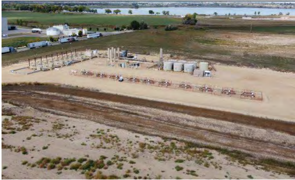
Oil and Gas Facility
